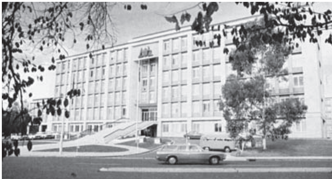
Treasury building, Canberra, housed the ATO Head office from 1969.
