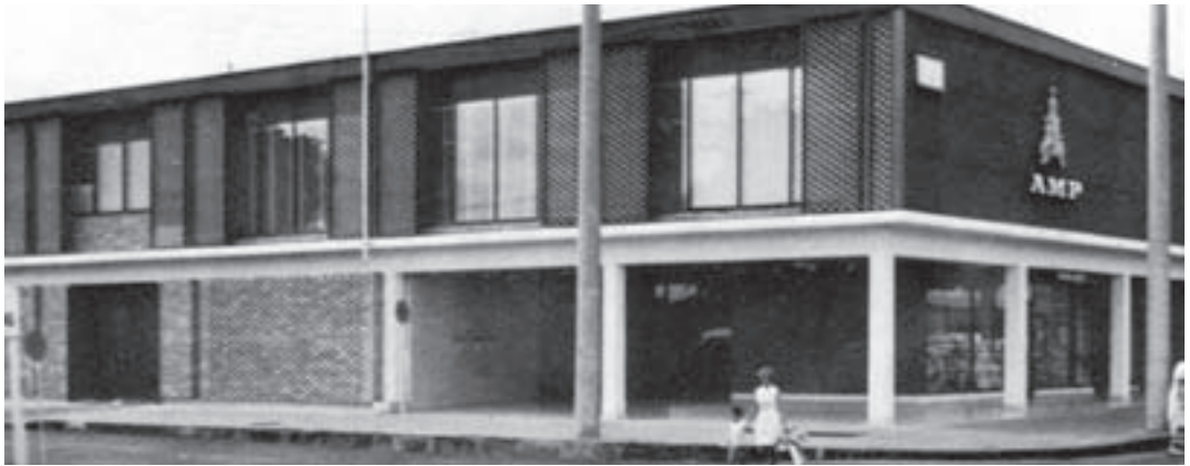
Lismore regional office, 1969. It was the first office in a predominantly regional area, situated about 800 kilometres from Sydney and serving about 12,000 residents.
