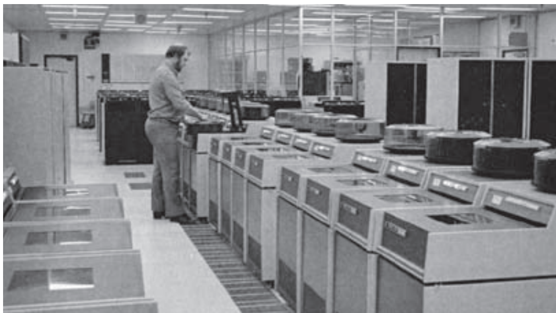
The central computer room, Canberra, 1985.
