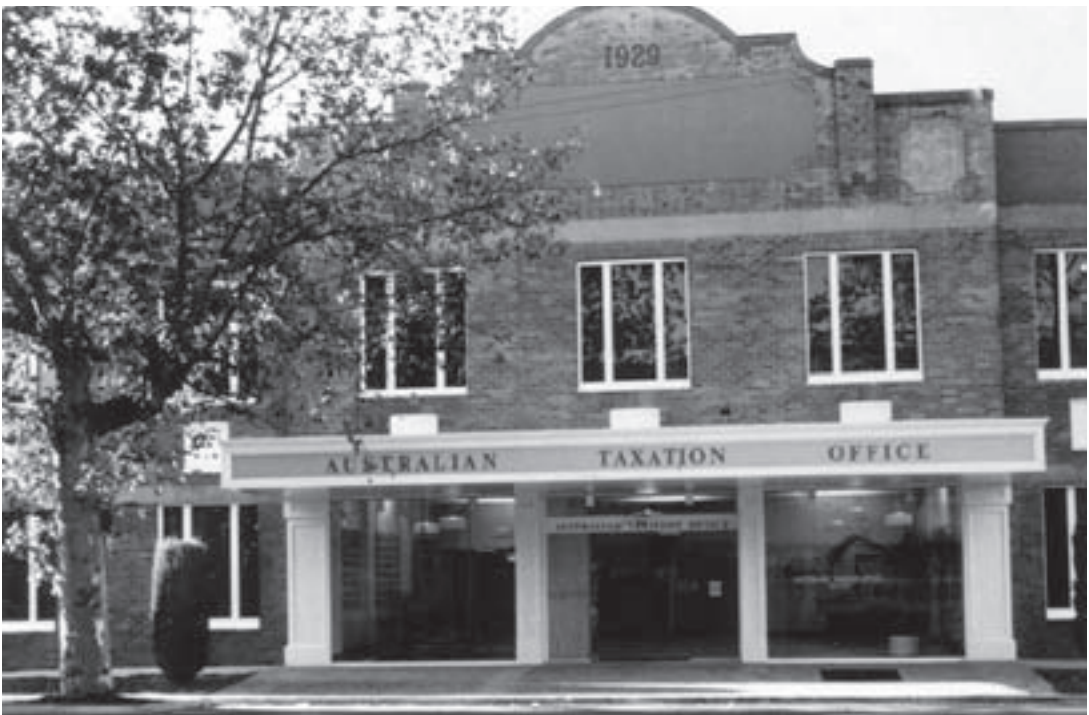
Albury-Wodonga branch. Most new ATO branch buildings were new but this branch was located in a restored wool store in central Albury.
