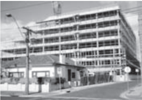
Moonee Ponds office under construction.
