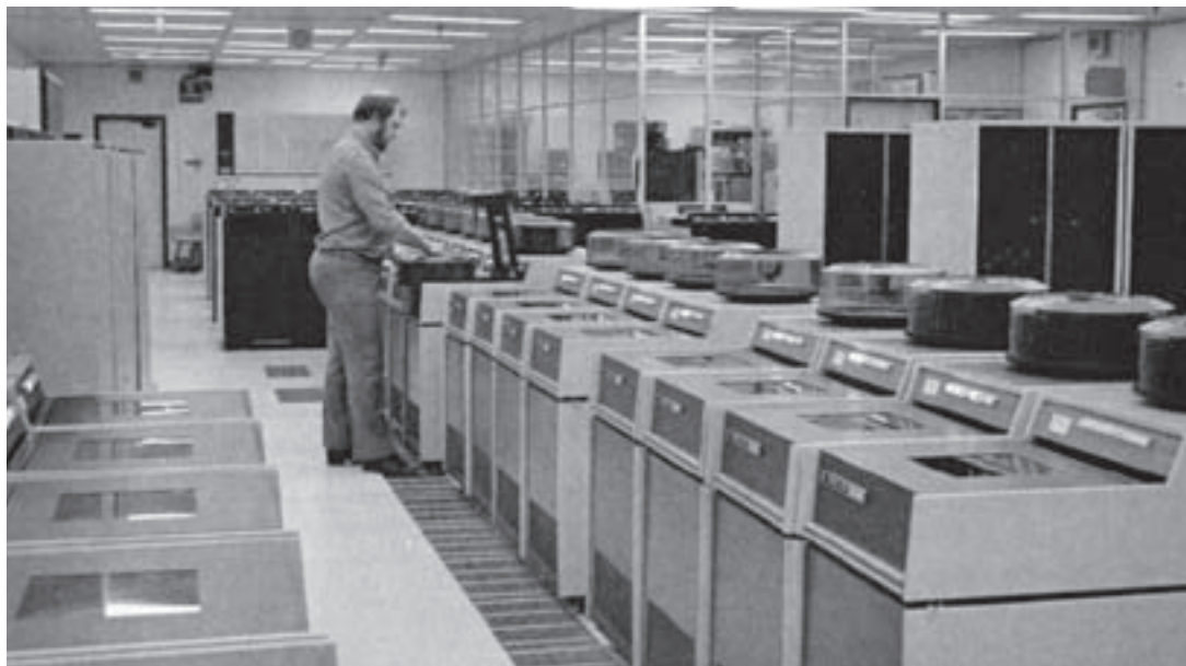
The central computer room, Canberra, 1985.
